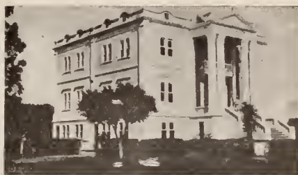
Main Building of the "Instituto Evangelico," Lavras, Brazil.
